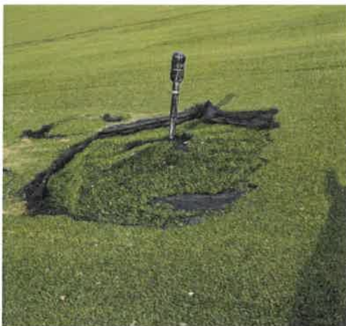
Photo 3 – Bird Damage of Engineered Turf Around Passive Relief Vent (PRV)
