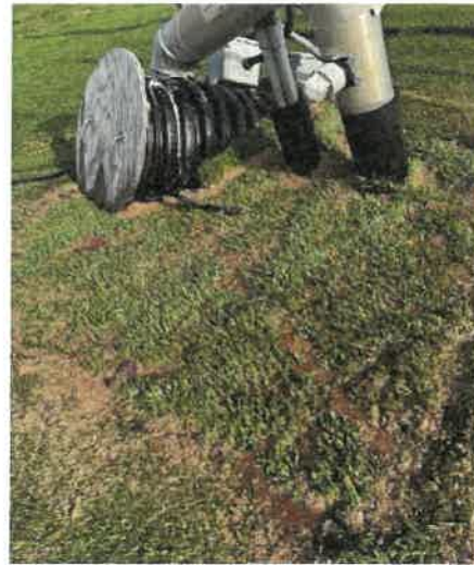
Figure 10. Repaired wrinkles and torn ClosureTurf® at leachate piping on south slope
