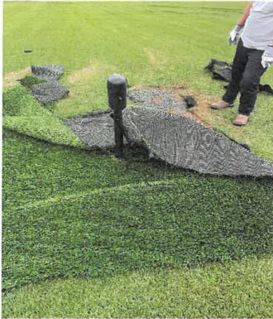
Figure 3. Repairing bird damage around PRV
