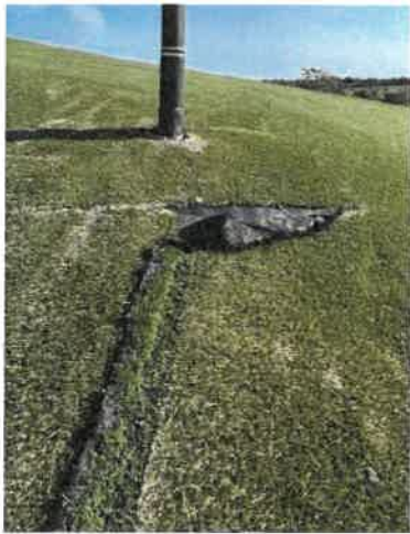
Figure 7. Bird damage at gas well
