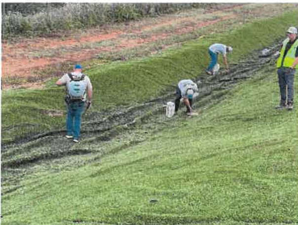
Figure 5. DuraGuard® and infill application to wrinkles
