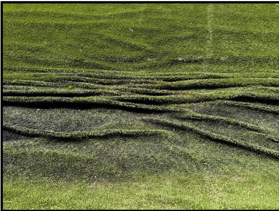
Photograph 6: View of coating added to closure turf wrinkles on north side Area 1-2.
