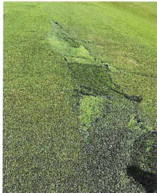
Figure 2. Bird damage at previously repaired location
