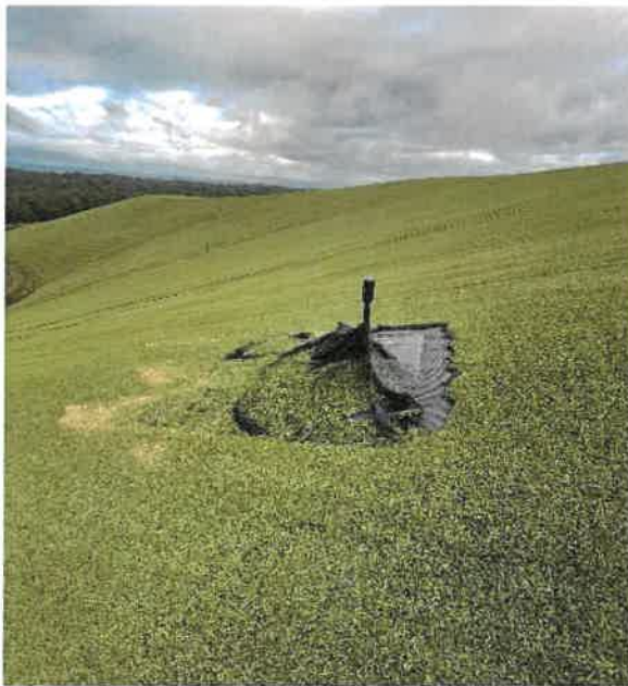
Figure 1. Bird damage around PRV
