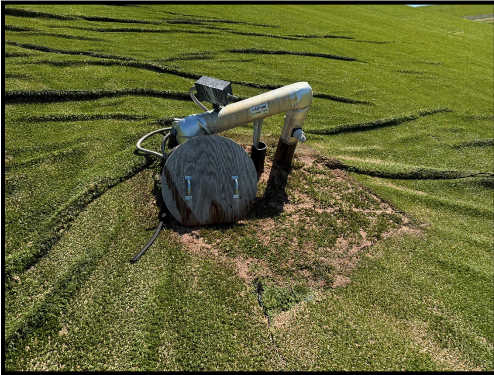
Photograph 5: View of closure turf repair at LCS-4 sump.
