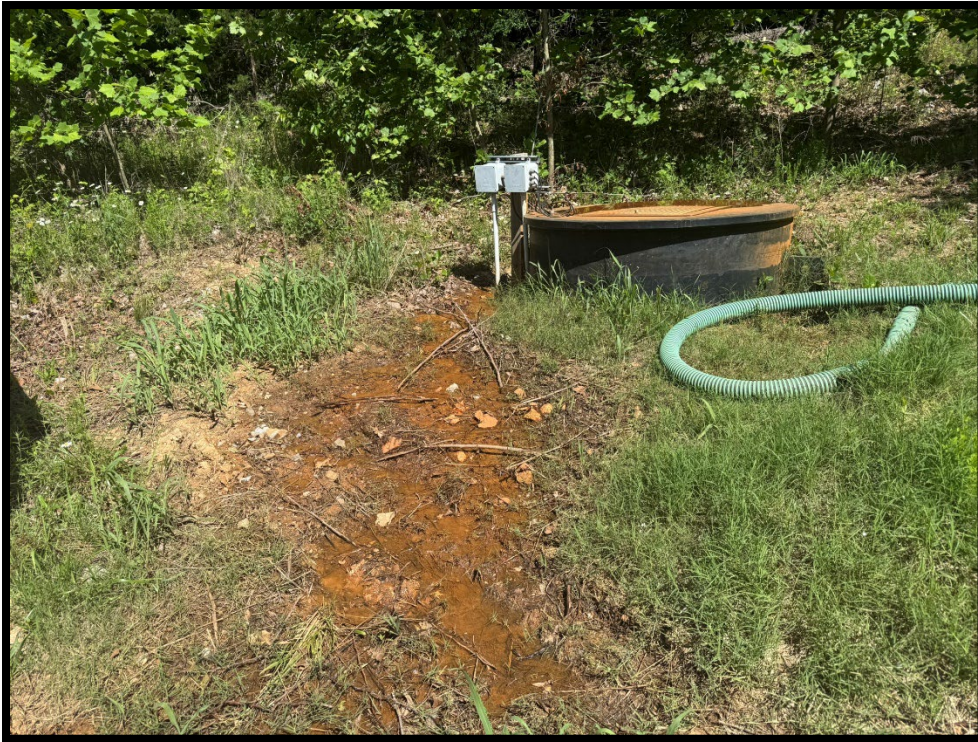
Photograph 1: View of erosional rill from VLCS-1 overflow.
